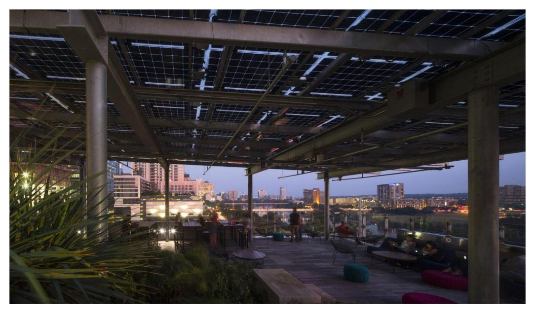
A photovoltaic cell generates 13% of the building's power and shades the rooftop garden. The Library uses 40% less energy than a building of comparable size.
