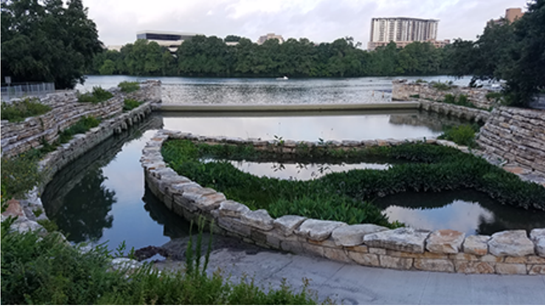
The Waller Creek Tunnel releases floodwaters into Lady Bird Lake at this outlet facility.
